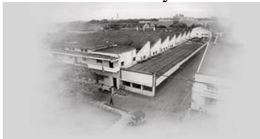
The factory at Tiruvottiyur, near Madras
